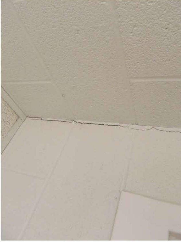
New cracks developing in CMU walls
