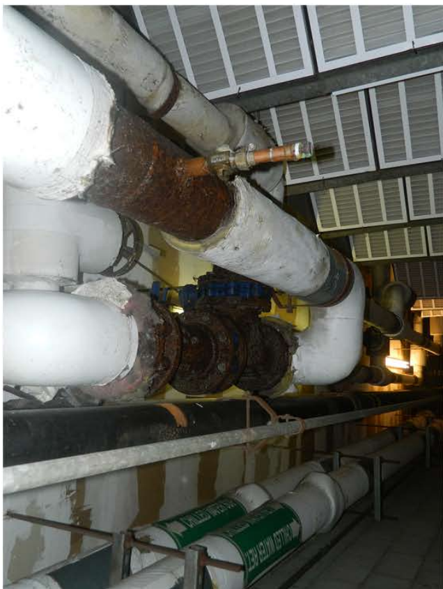
Rusted piping where damaged insulation was removed.
