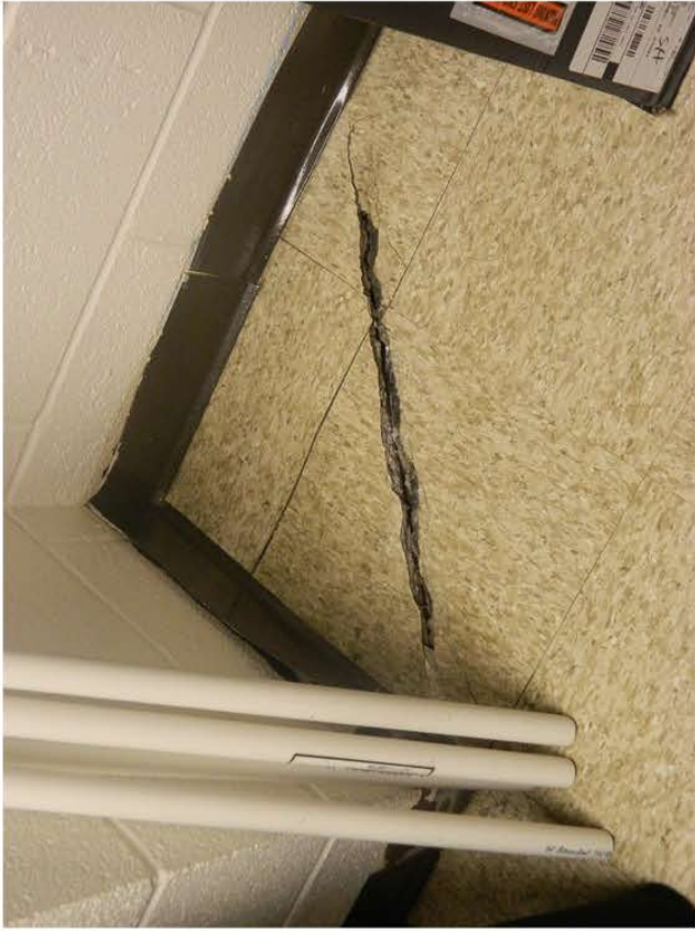
Concrete Cracking and settling
